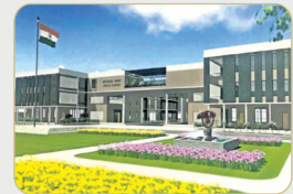
RR Dist. Collector Office - 25 Mins
